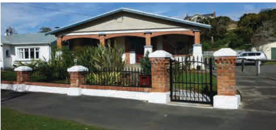
The Georgia design pedestrian gate shown here with non standard arch top fence panels completes the fence of this solid brick bungalow
